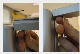
**3.** When positioned, tighten widget to secure in place
